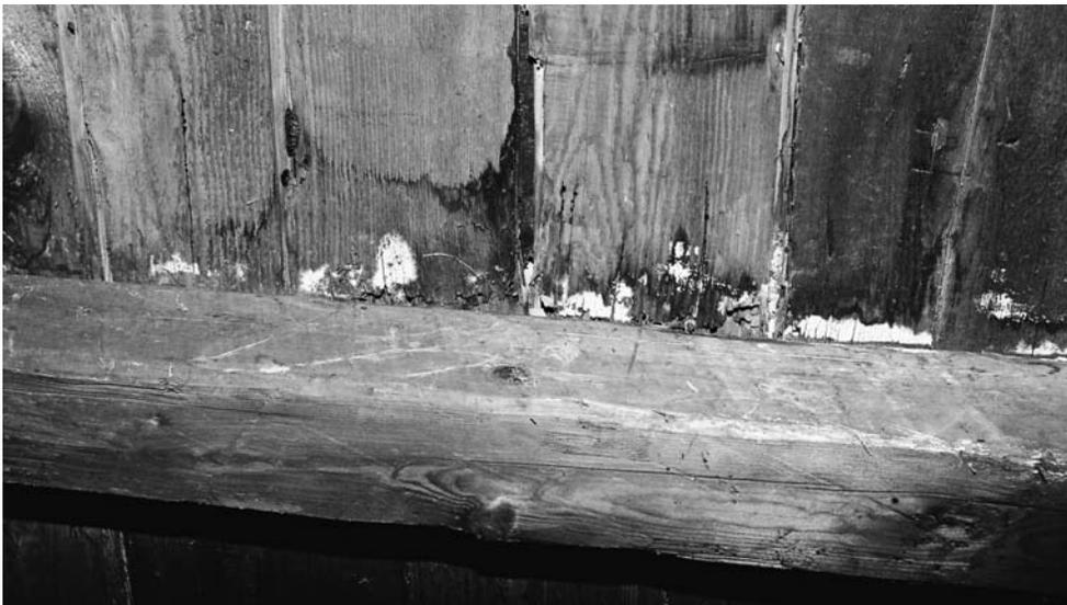
Fig. 5. The wooden roof of the outside room damaged by *Athelia decipiens*.
