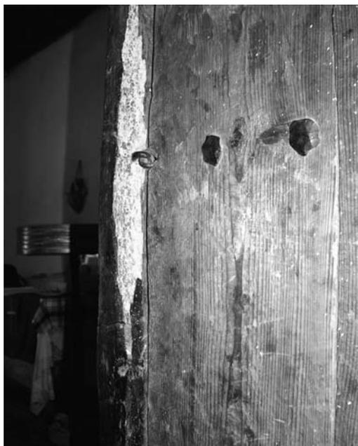
Fig. 3. Inner door with fresh damage of Anobiidae insects.
