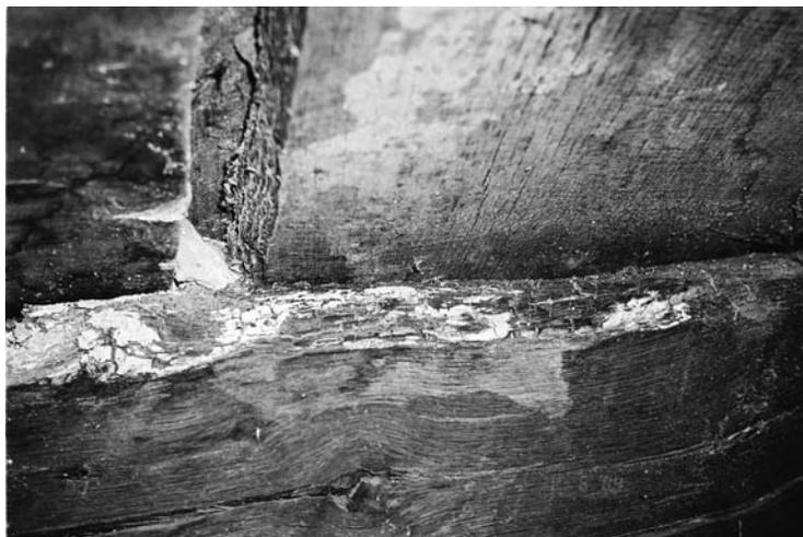
Fig. 6. Roof construction attacked by *Hyphodontia crustosa*.
